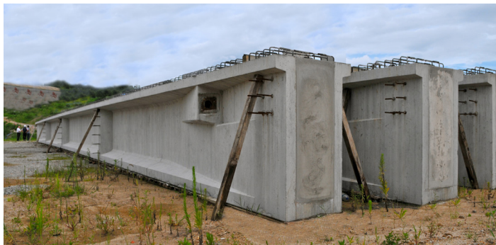
IPC _ Incrementally Prestressed Concrete Girder
