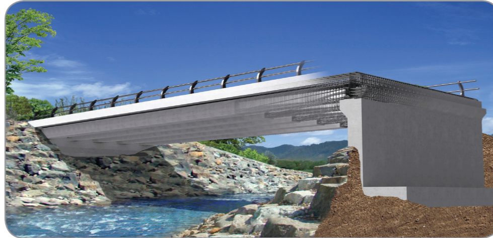
Spliced PSC Box Type Rahmen Girder
