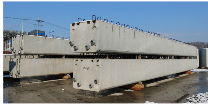
SegBox _ Spliced PSC Box Type Girder
