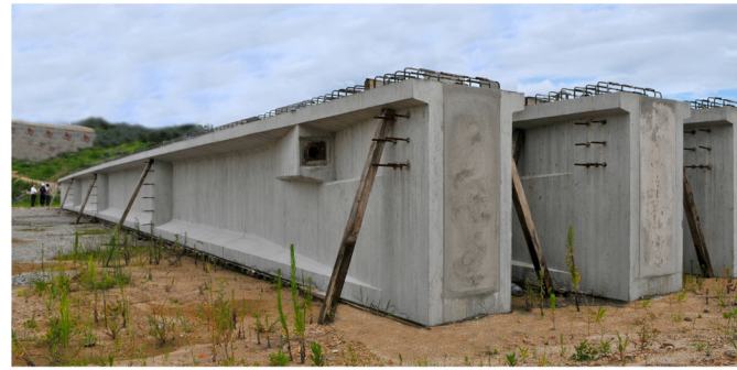
IPC _ Incrementally Prestressed Concrete Girder
